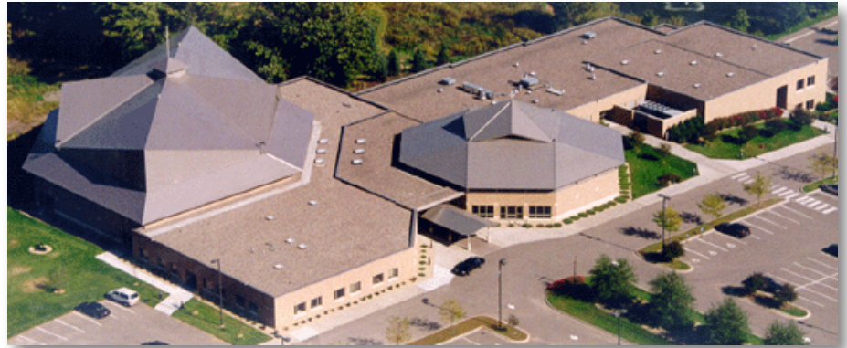
St. Andrew Lutheran Church, Eden Prairie, is the setting for the 2011 Synod Assembly.
